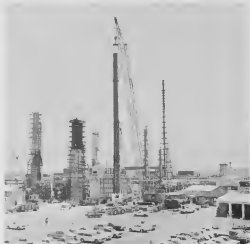
The L2AR's 150-ft stack is back in place against its furnace following refractory lining to its interior.
